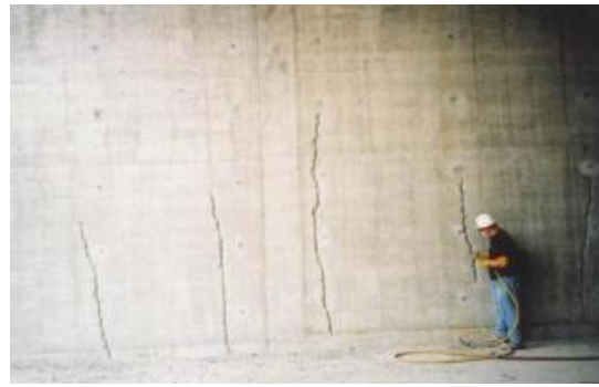
Figure 2.4 Repairation of shrinkage cracks in a wall. b
