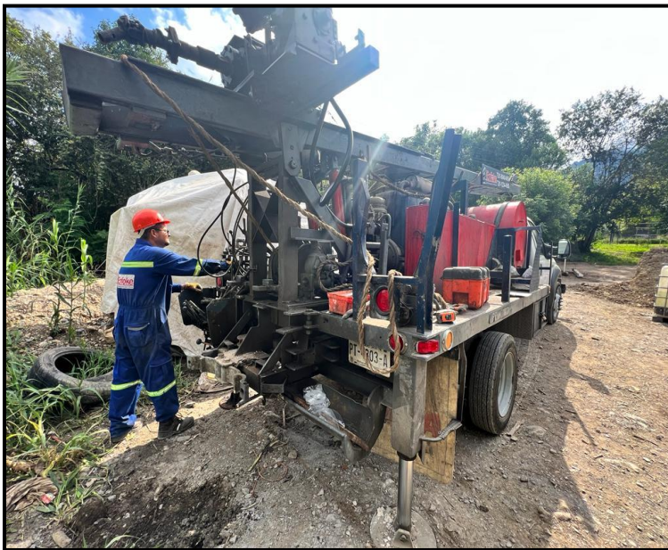
Figura 1. Perforadora Mobile Drill B-50.
