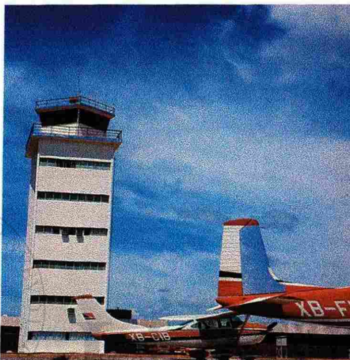
Fig.9.1 Torre de control
