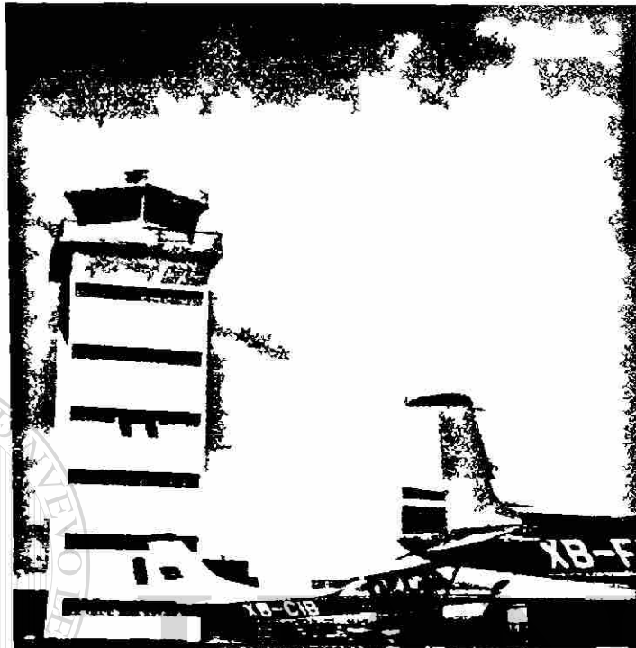
Fig.9 1 Torre de control
